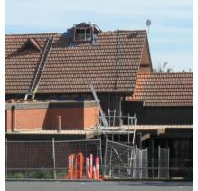
On Tuesday 23<sup>rd</sup> April the terracotta tiles were put back on the section of roof where the steel base framework has been installed. The internal wood panel work of the ceiling has also been put back in place, concealing the steel framework. The removal of the scaffolding from inside the Church has been delayed till this week.
