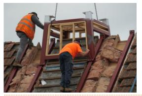
Scaffolding will remain in the Church through this week and will be removed early the following week. The next steps will be putting the tiles back in place on the roof, and then the cladding with zinc of both the base and the steeple. A large cross will surmount the whole structure once the steeple is lifted into place. The bell will be added later in the year with a formal blessing.
